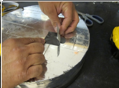
Fig. 23. Septa held in place with tape.
